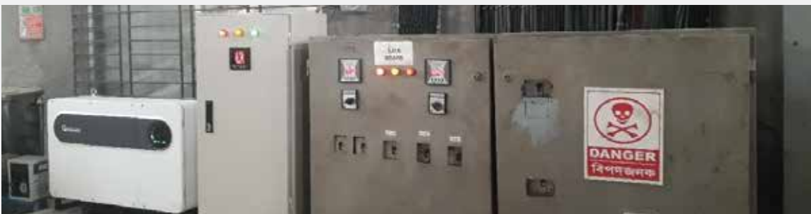
SOLAR ON GRID INVERTER INSTALLATION
