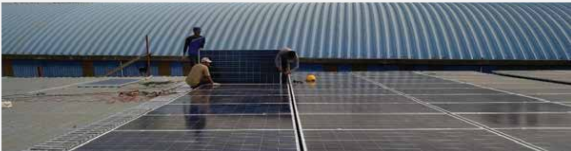
SOLAR PV MODEL INSTALLATION
