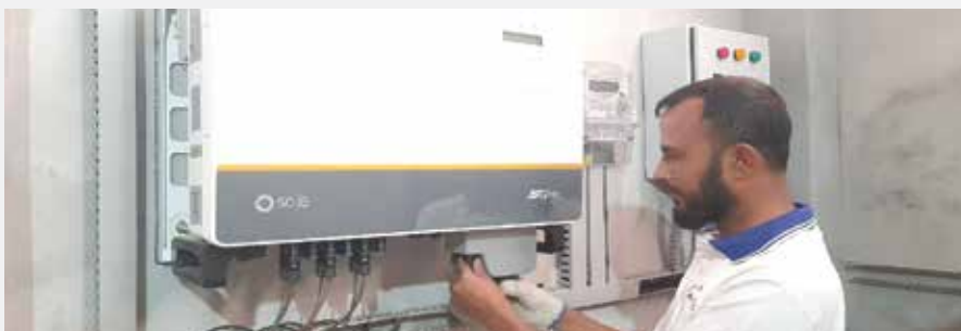
Inverter Installed
